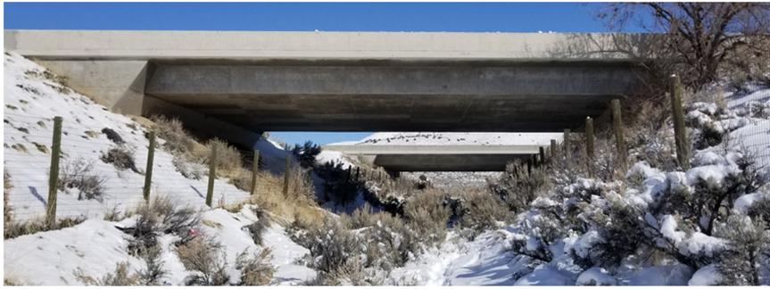
**Figure 2.** One of 3 highway underpasses on United States Route 395 in Hallelujah Junction Wildlife Area, California, USA, February 2019. The underpasses all had a similar structure, with an open atria in the center and fencing on the sides. The underpasses were approximately 120 m in length, 5 m high, and 6 m wide.
